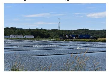
The ecology in the second pond is very different than the first. Generally free of sludge, it looks and behaves like a water body found in nature. Commonly called the "finishing pond", aerobic microbes ingest remaining nutrients in the water column, resulting in a clean, clear, polished effluent that can reenter our environment. The second ponds in our municipality are commonly filled with ducks, geese, turtles, muskrats, and duckweed.
